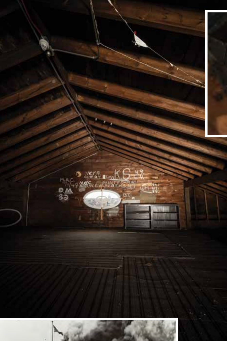
Blackened rafters and beams in Bascom Hall's attic trace how far the 1916 fire reached.
